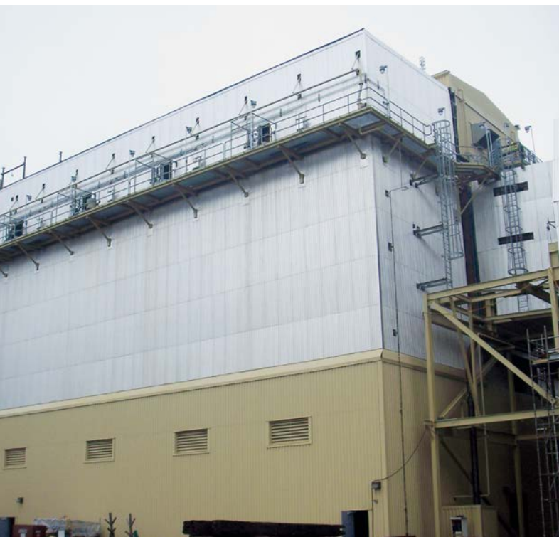
B&W successfully converted one of the two 300 MW electrostatic precipitators on a 600 MW coal-fired boiler into a single-casing pulse jet fabric filter serving the entire boiler.
