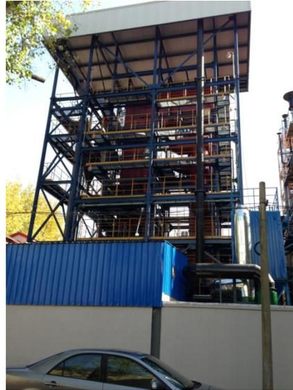
**Figure 6.** Pilot Plant 2.5 MW<sub>th</sub> Pilot Plant with U-Beams and IBHX
